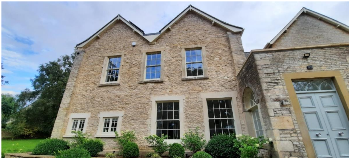
The current view of the house if looking towards the church. This was an original internal wall, which became an external wall in 1937. The house's original windows were reused in this renovation.
